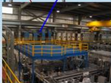
TITAN platform finished at ISAC
