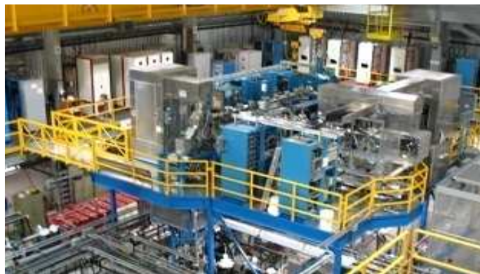
Fig. 2 TITAN platform in the ISAC I experimental hall
